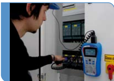
Magnetic holder for hands free operation
